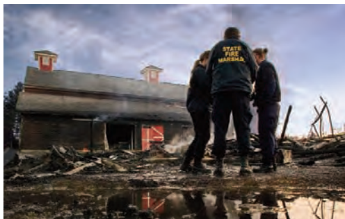
Aftermath of the fire at the Weathervane Theatre. (Photo: Mark Winter)
